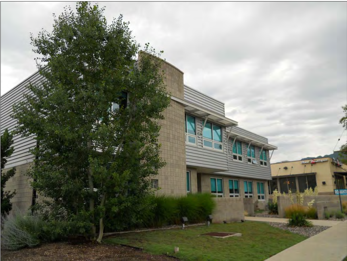
Adjacent Block Face East of Development – 1371 E 2100 South
