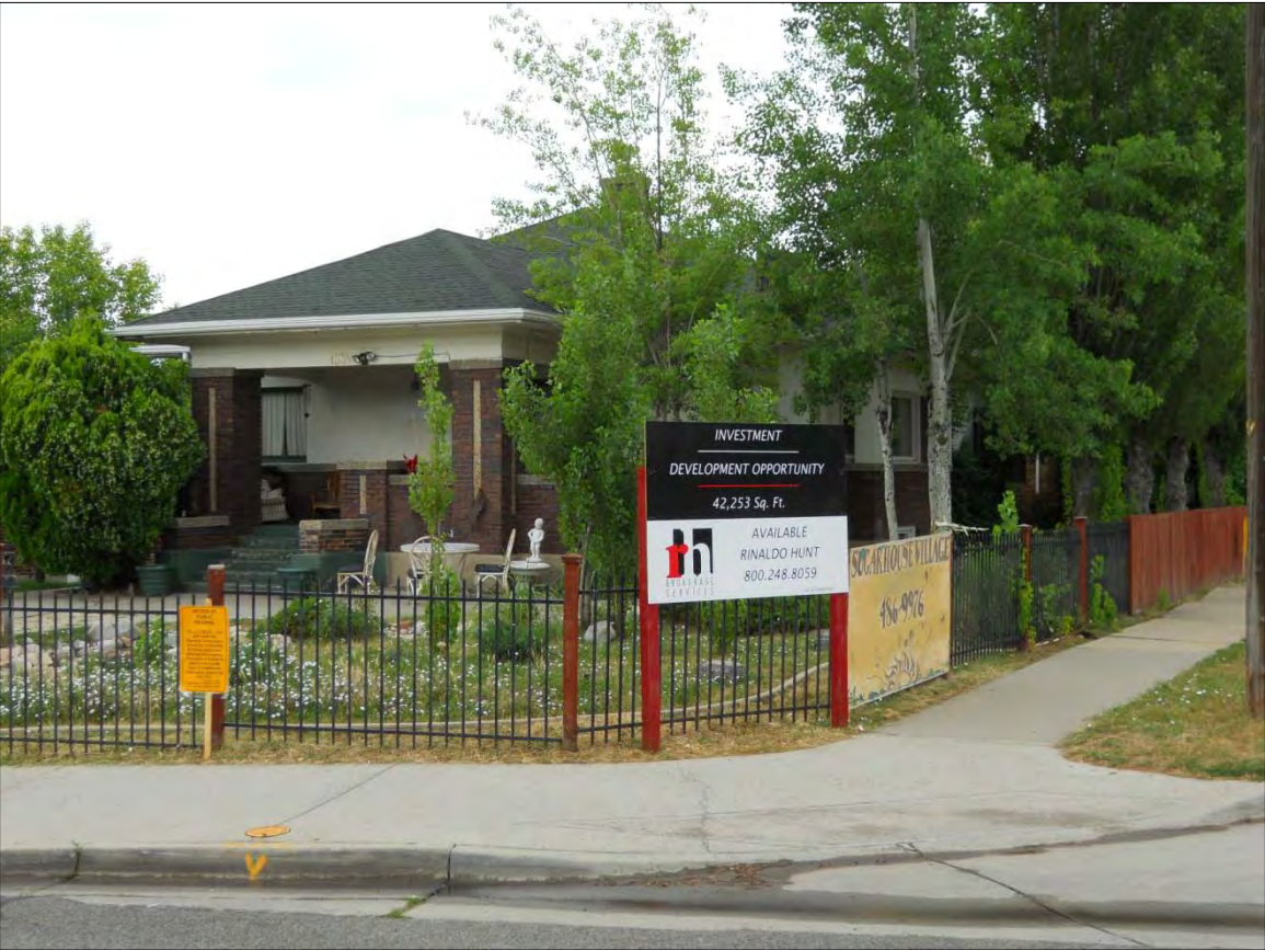
Corner Parcel Located at 1339 E 2100 South
